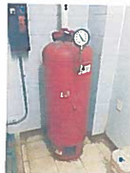
WVNCC - Wheeling Expansion Tank 402
