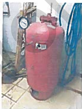
WVNCC - Wheeling Expansion Tank 401
