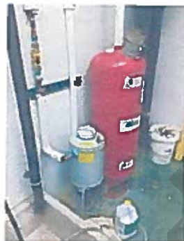
WVNCC - Wheeling Expansion Tank 201
